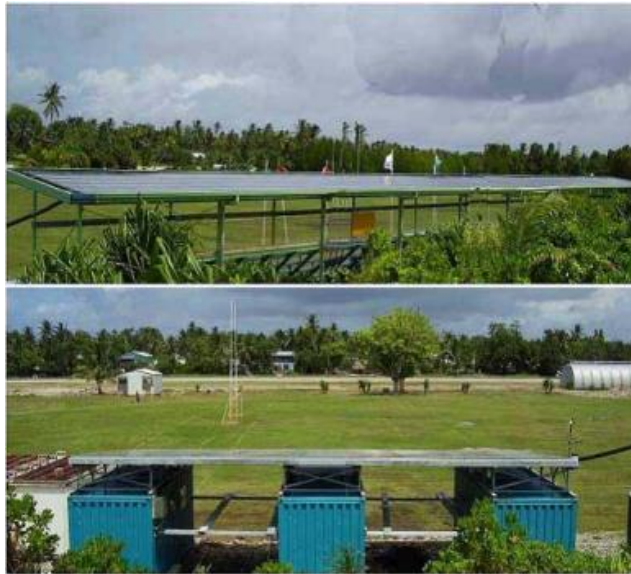
40kW solar PV grid-connected system at the football stadium in Funafuti
