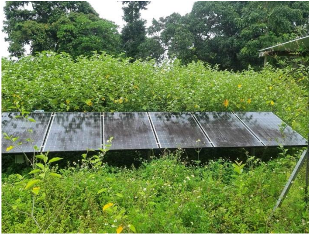
Houma SWP site showing the overgrown bush shading the PVs
