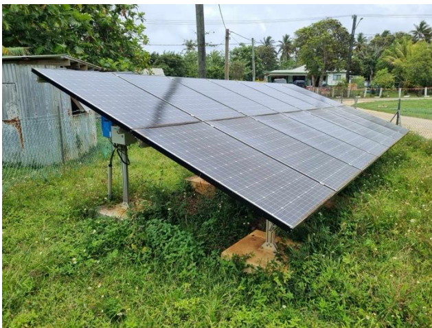
Pangaimotu solar water pump system
