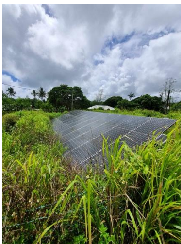
Leimatu'a SWP site showing the overgrown bush shading the PVs
