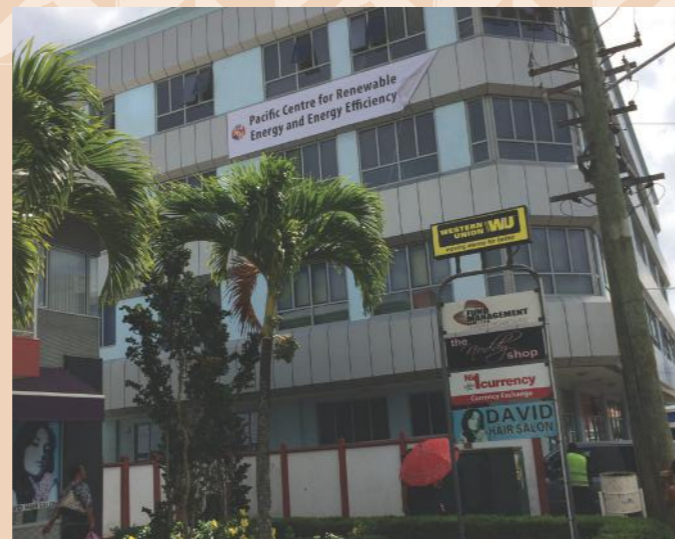
The PCREEE Office at the Third Floor of O. G. Sanft Building at Nuku'alofa
