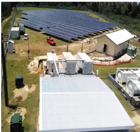
Picture 3. Ha Mai Solar Facility on the island of Ha'apai – the first island in Tonga to reach 50% renewable energy (Tonga Power)
